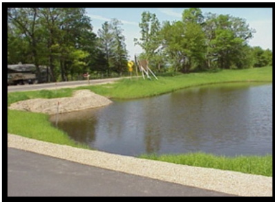
Stormwater retention pond
